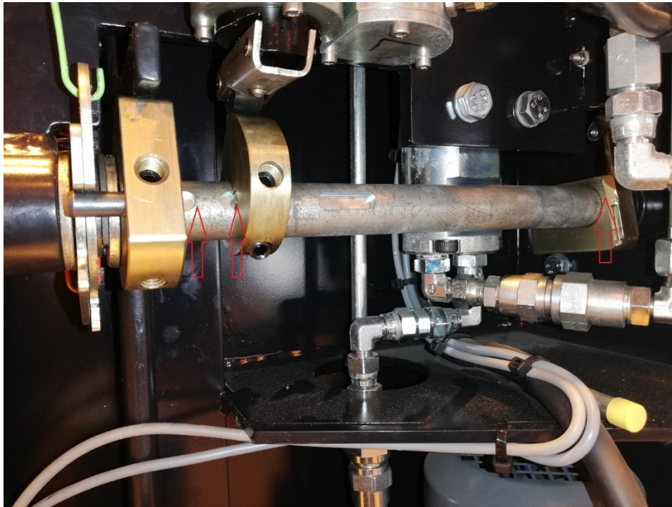
Picture 2 Door with keyway
